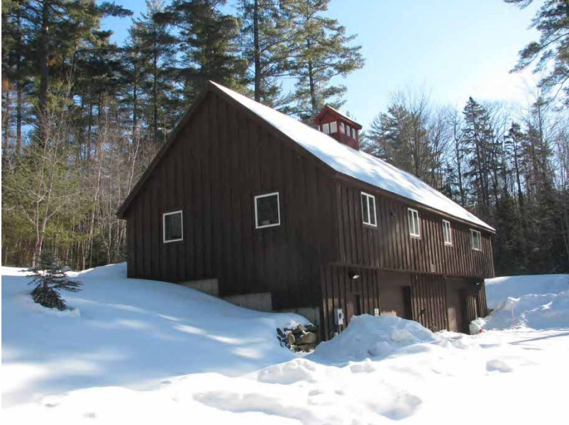
Ranger's residence/maintenance building on Little Pond Road
