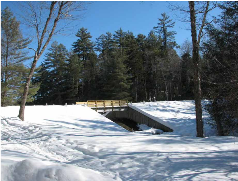
Lowell Lake dam and bridge
